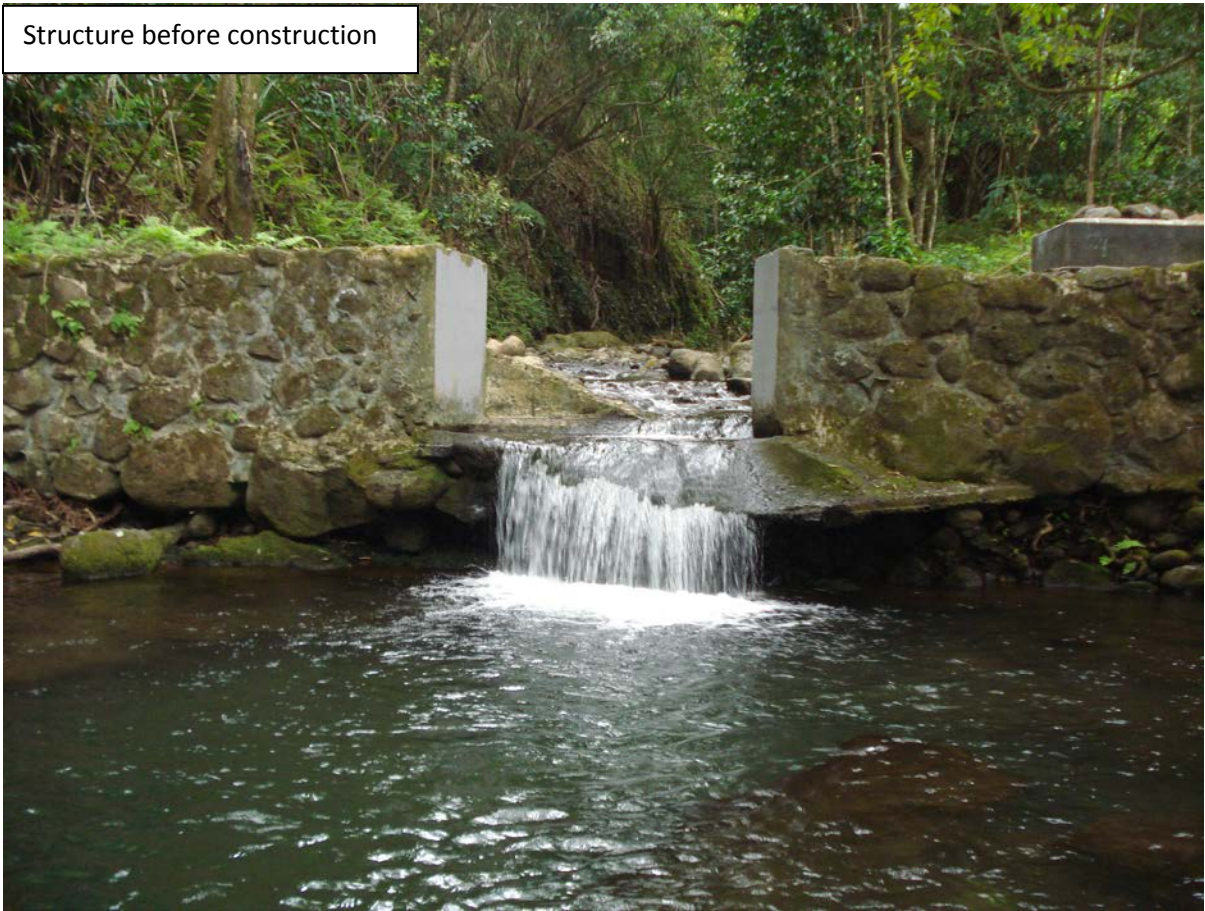
Phase I- Stockpiling rocks at site
