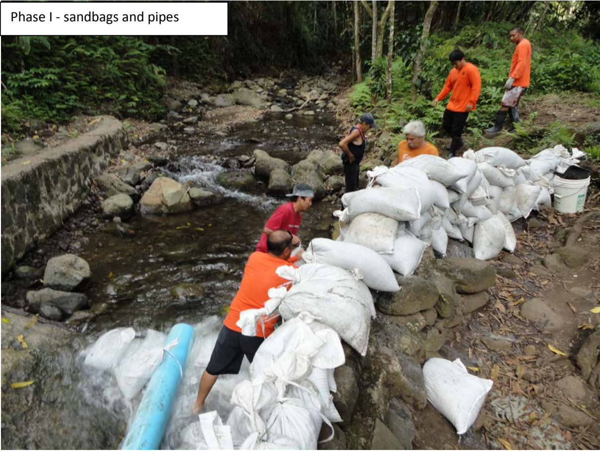
Phase I - sandbags and pipes
