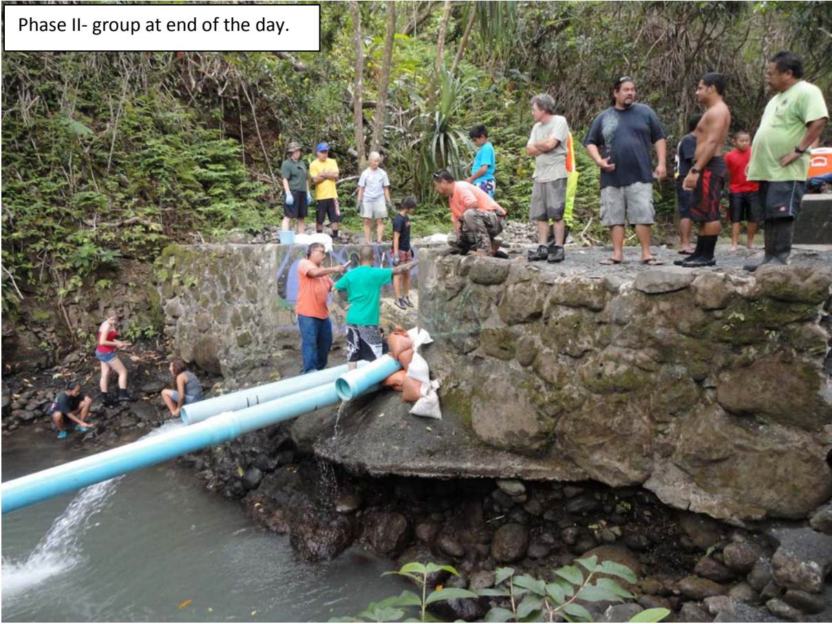
Phase II- Repairing the wall
