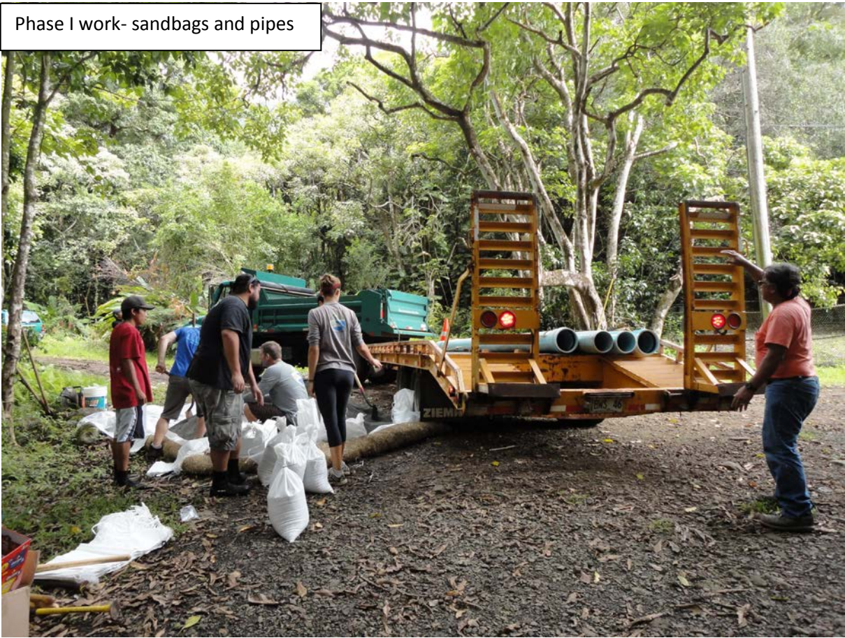
Phase I - sandbags and pipes
